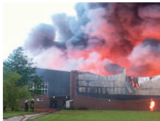
WAREHOUSE DEVASTED BY FIRE
